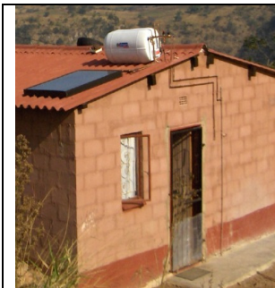
Solar Water Heater (100 litre) at Welbedacht R4,475 including installation
