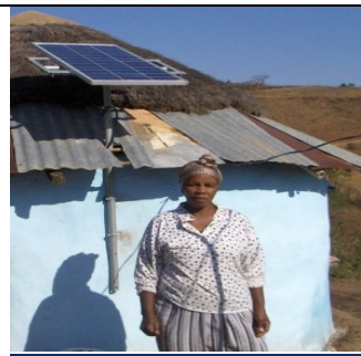
PV Solar Home System (65 Watt incl. battery & controller) at Dududu R4,266 including installation
