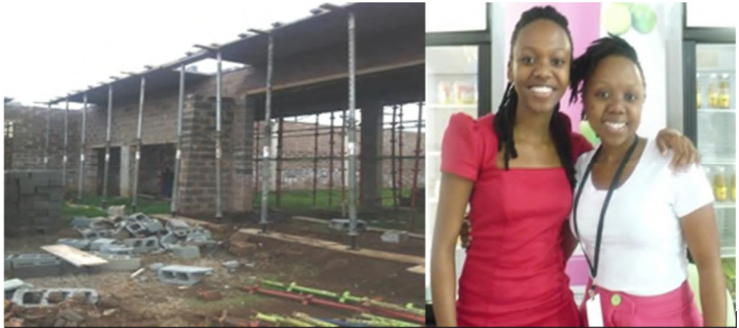
Frutee Belliez entrepreneurs Masibonga and Mbali alongside the construction site that is now their new factory in Waterfall, eThekweni. The enterprise's core business is preparation and packaging of vegetables and fruit.
