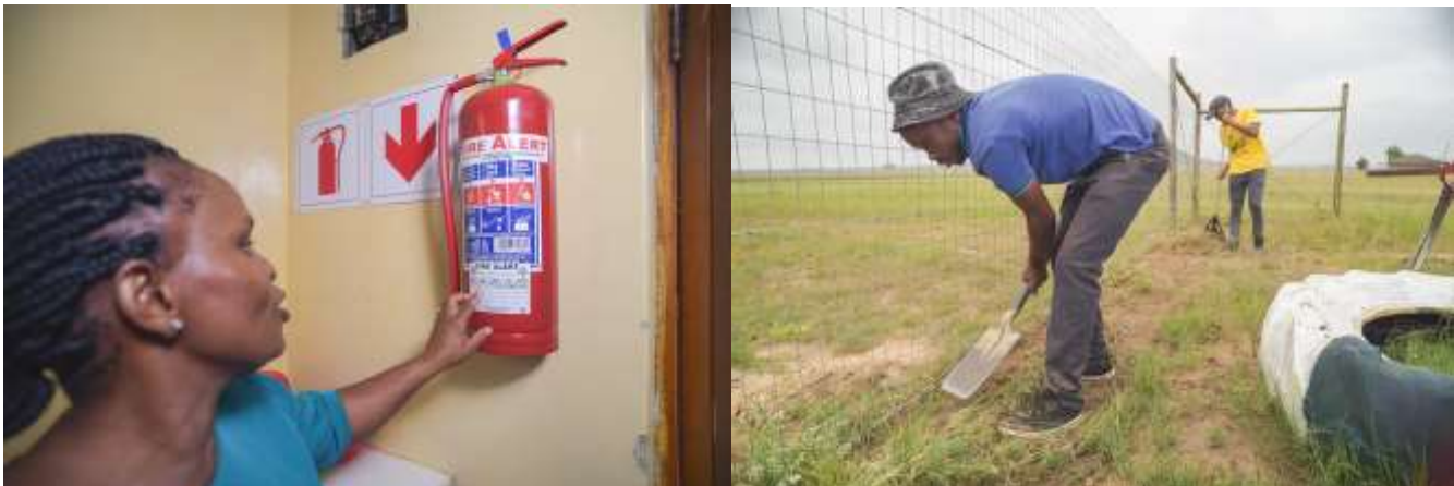
Figure 10: Fire extinguisher and signage
