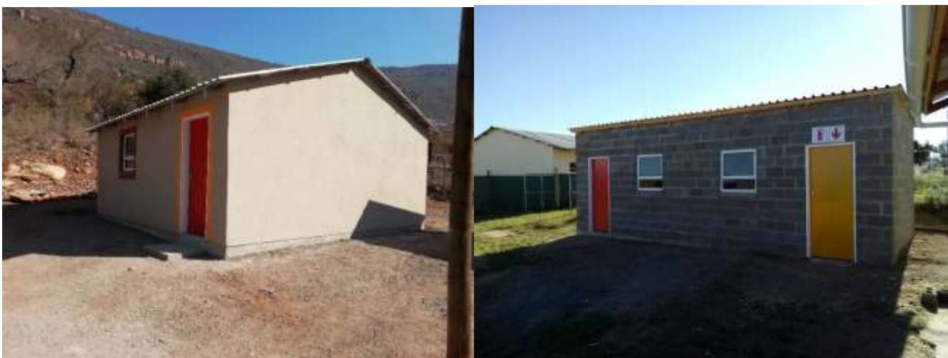
Figure 5: Additional classroom at Sibusisiwe Additional office and kitchen at Thandanani
