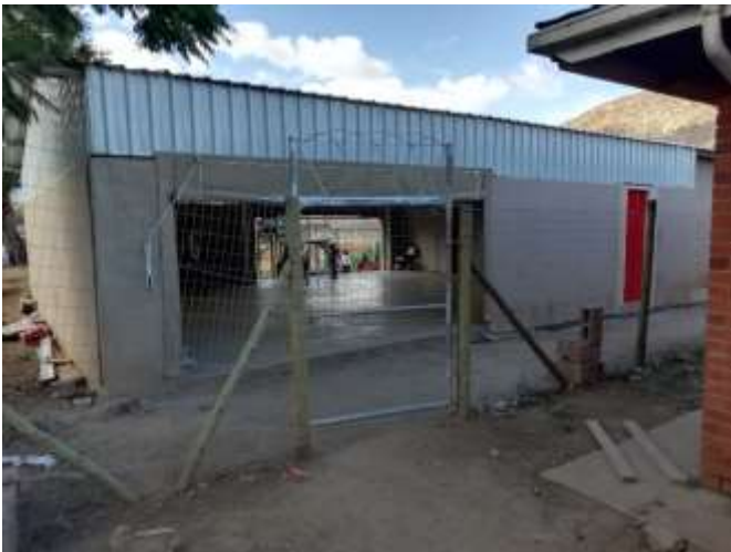
Figure 7: Sinozwelo approaching completion
