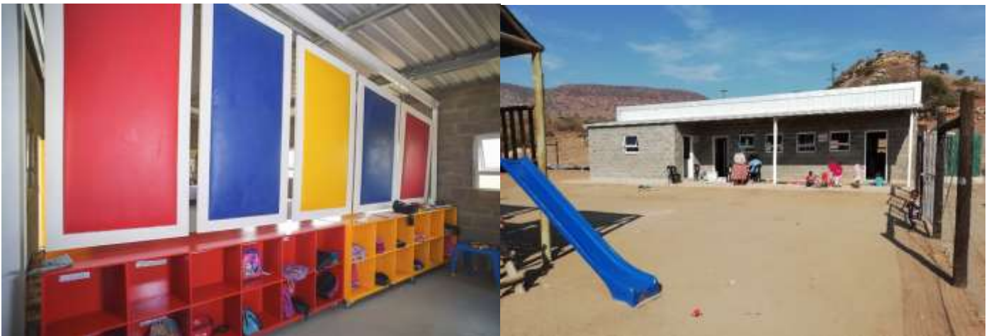
Figure 1: Internal partitioning in progress
