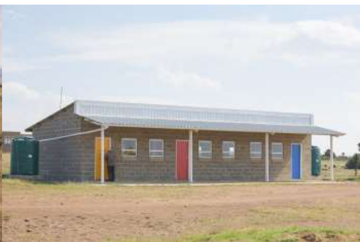
3 new classrooms at Qhapelani
