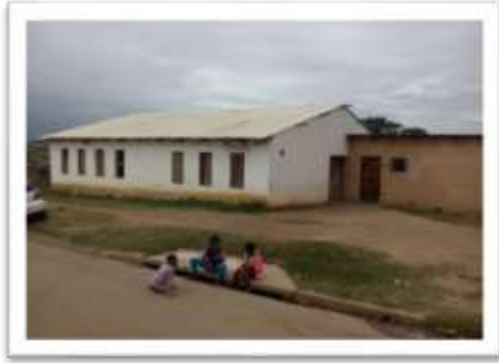
Example 1 - big structurally sound building
