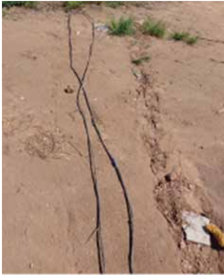
Electrical wires strung across a road.
