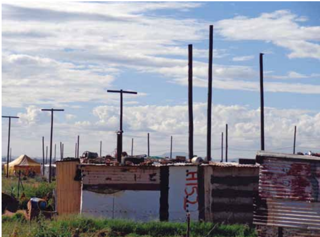
Electricity poles in Dinaweng in preparation for electrification.
