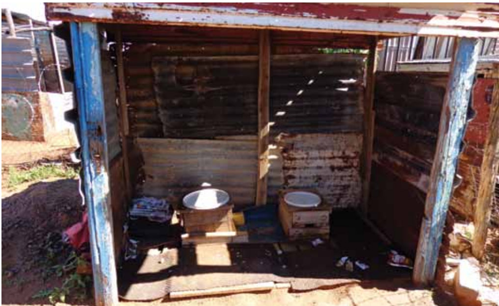
Pit latrines for children's use.
