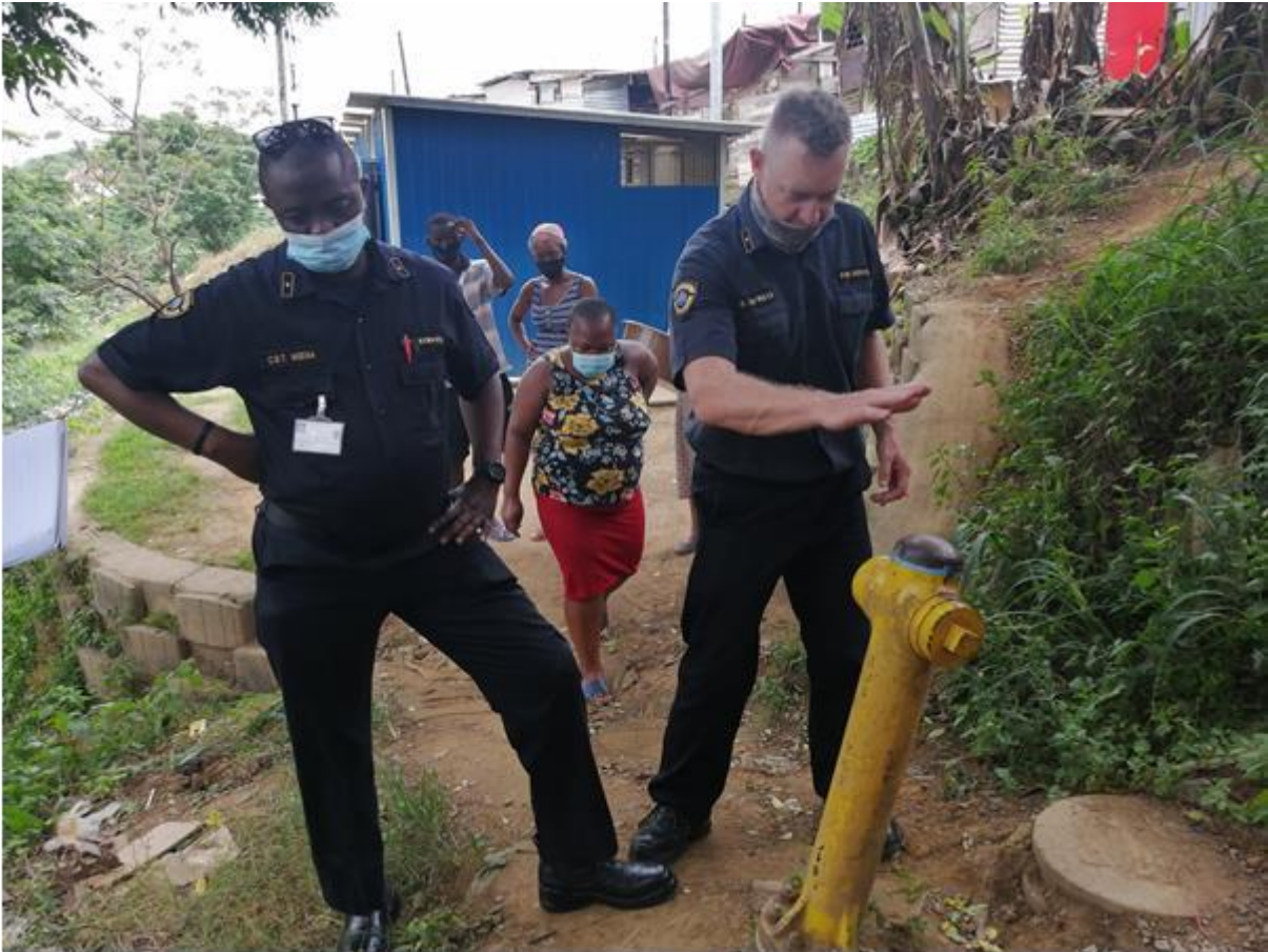
eThekweni Emergency Services personnel showing inaccessible fire hydrant in Parkington which renders fire fighters inefficient in adequately dealing with informal settlement fires.
