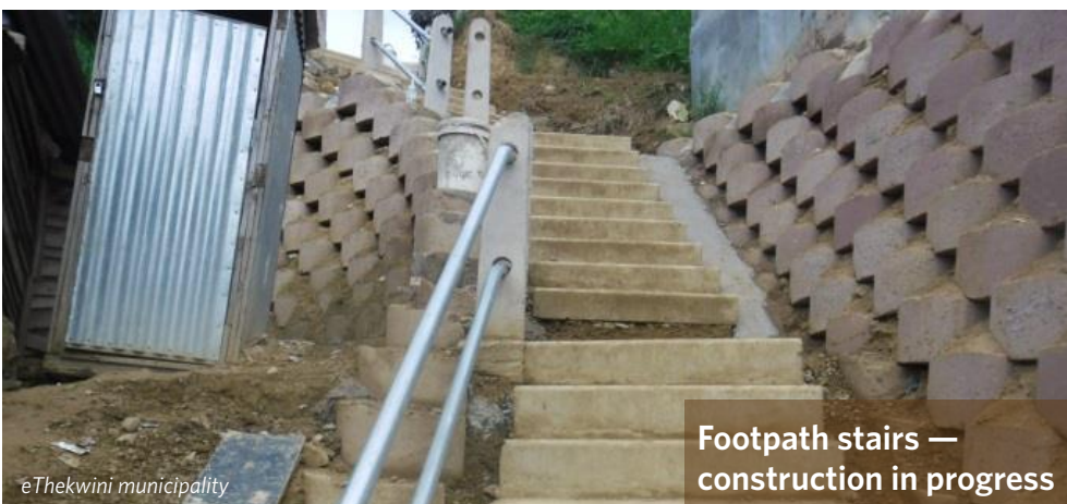
Foot path access — construction in progress
