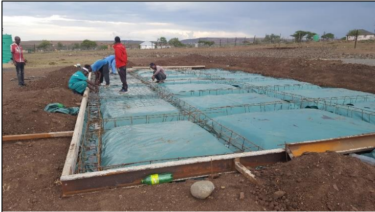
Nsukanghlale preparing foundation for pouring
