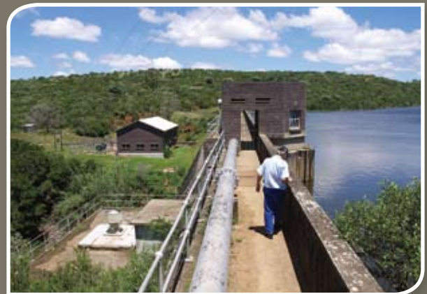
Howiesonspoort Dam and Pump Station.
