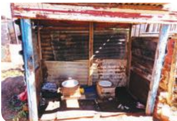
Pit latrines for children's use.
