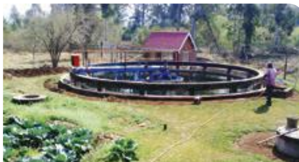
Richmond Waste Water Treatment Works Project: Through Ukulungisa, PPT successfully leveraged R21.1 million for the upgrading and refurbishment. Ukulungisa funded feasibility work and an application for capital funding from the Municipal Infrastructure Grant (MIG).
