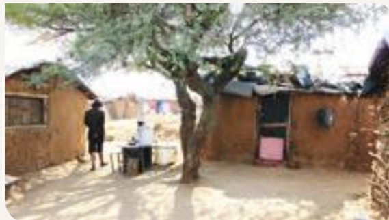
A central yard and communal meeting place within the Thokoza informal settlement are approximately 80 families in the settlement that is serviced with only one yard tap and informally constructed pit toilets. The rapid provision of basic services is a high priority.
