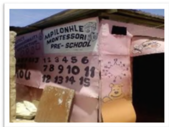
Photo 3: Informal corrugated iron structure
